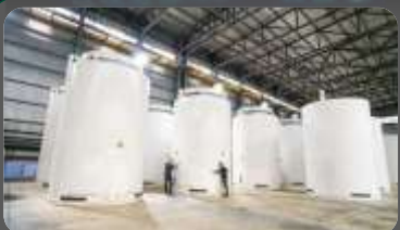
Langtidslagring indkapslet i 50 cm beton. Sizewell Spent Fuel Cannisters, UK
